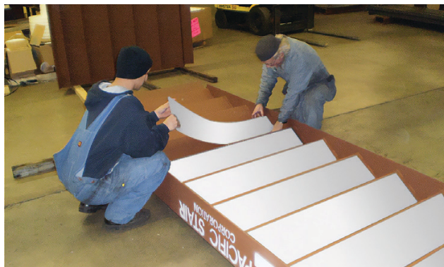
Shop Install on the underside of new metal stairs
